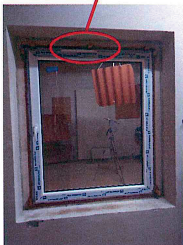
From receiving room side
