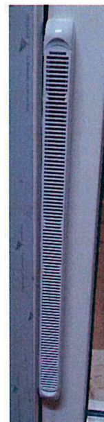
Fig. 4b. Photos of window with air intake system made during the test
